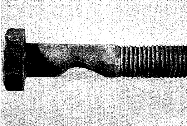
Figure 28. Shank of bolt showing crevice corrosion of shank at area of bolt where it was in contact with a flange and gasket.
