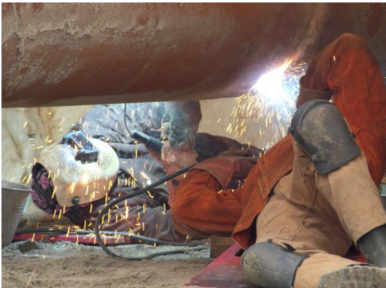
Pipe line welders
