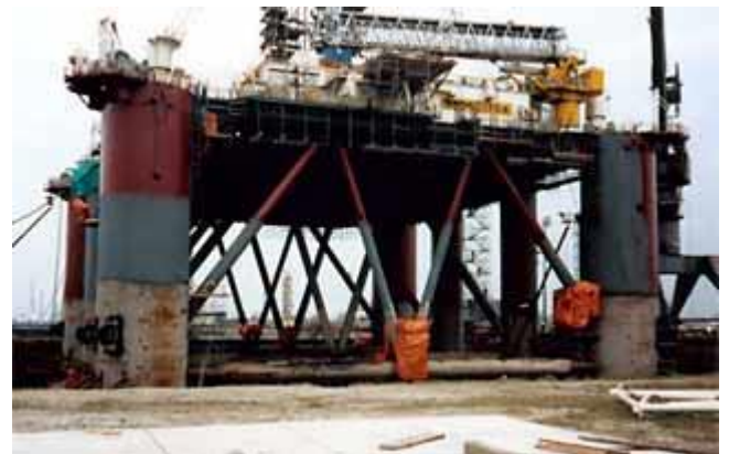
Platform in prefab fase.
